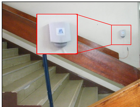
Figure 10. Plate Antenna placed at an entrance/exit point
